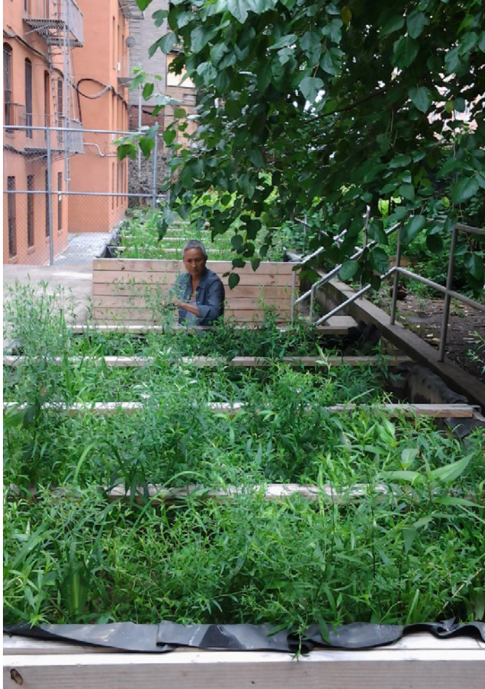
Stormwater Planters, 1203 Fulton Avenue, Bronx, New York Property owner: Community Assisted Tenant Controlled Housing (CATCH) Design & Engineering: eDesign Dynamics Project Lead: NYC Soil & Water Conservation District (Courtesy of NYC Soil & Water Conservation District)
