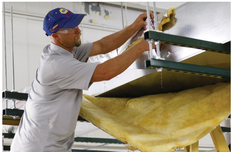
SOFT® Duct Wrap FRK fiberglass blanket being installed.
