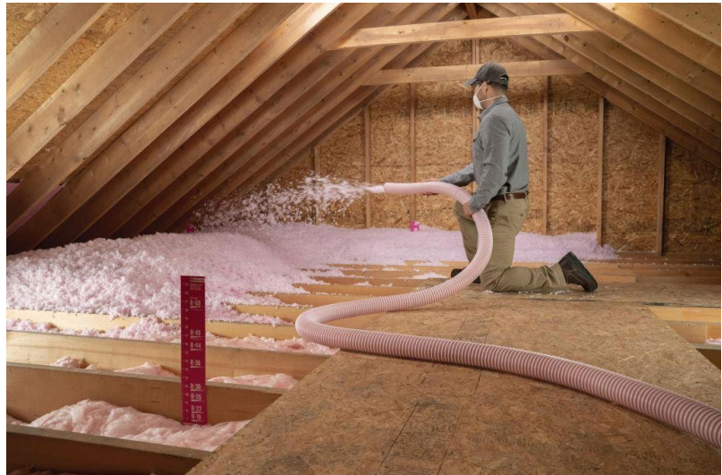
AttiCat® PINK® Blown-In Insulation installed in an attic.
